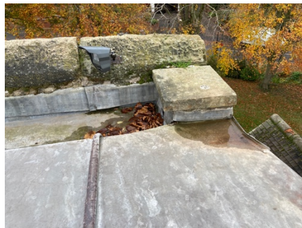
New alarm device
