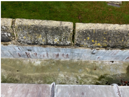
Open joint north side
