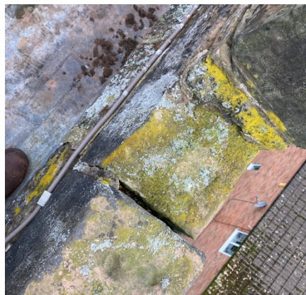
Open joint north side
