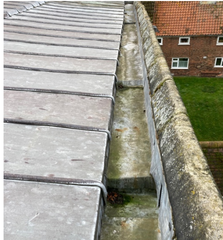
Clear, well stepped gutters
