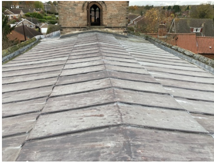
Nave roof leadwork
