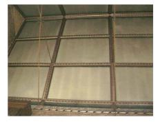
d It has been reported that grit is falling from high level at the west end of the chancel – this could be an indication of some loosening joints or friable. A closer inspection is advised if access can be arranged
