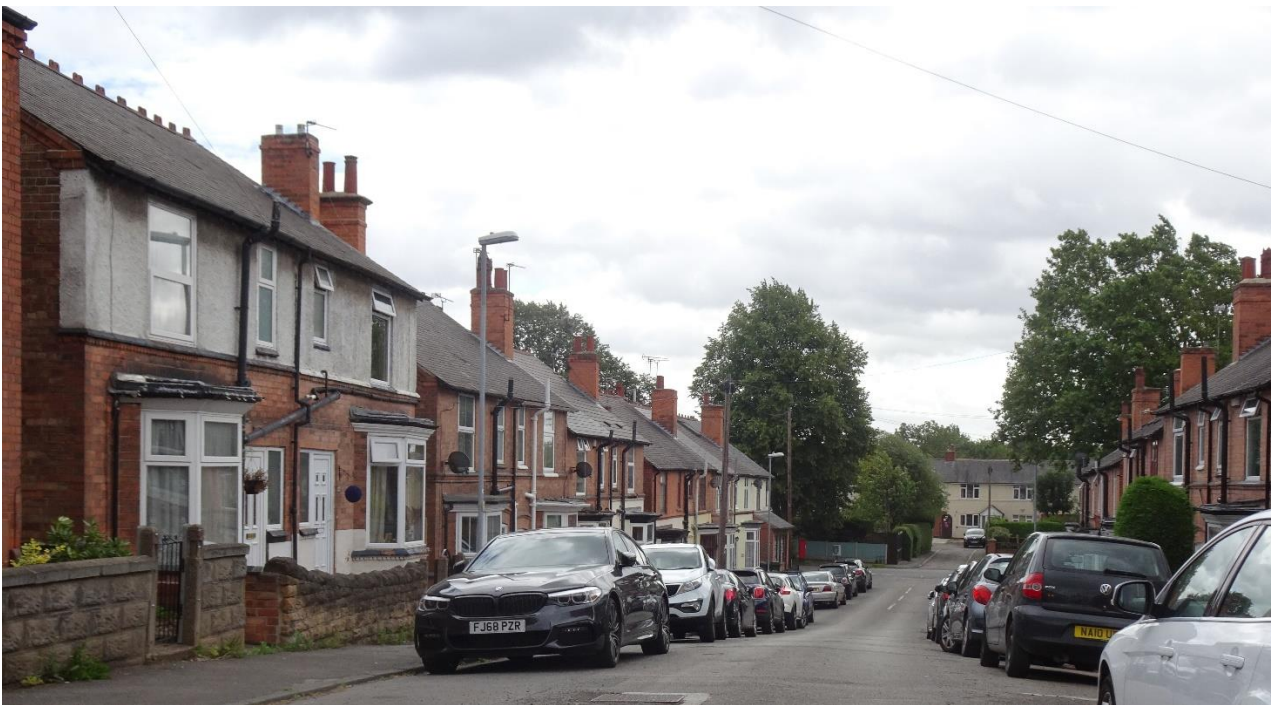
Willow Road looking towards Conway Road. Number 27 is on the left Photographed in 2020
